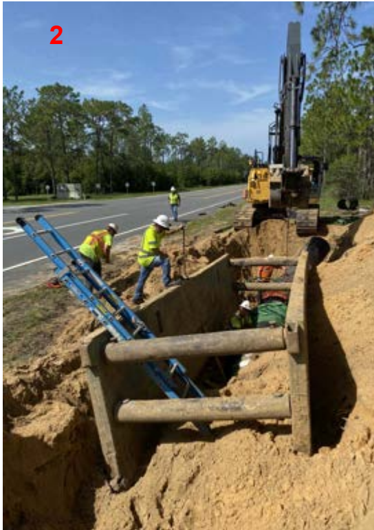
THE SR 21 PIPELINE: Above, the pipe installation has reached Gold Head Branch State Park! On the right, the pipe has been run in the casing under SR-21.
